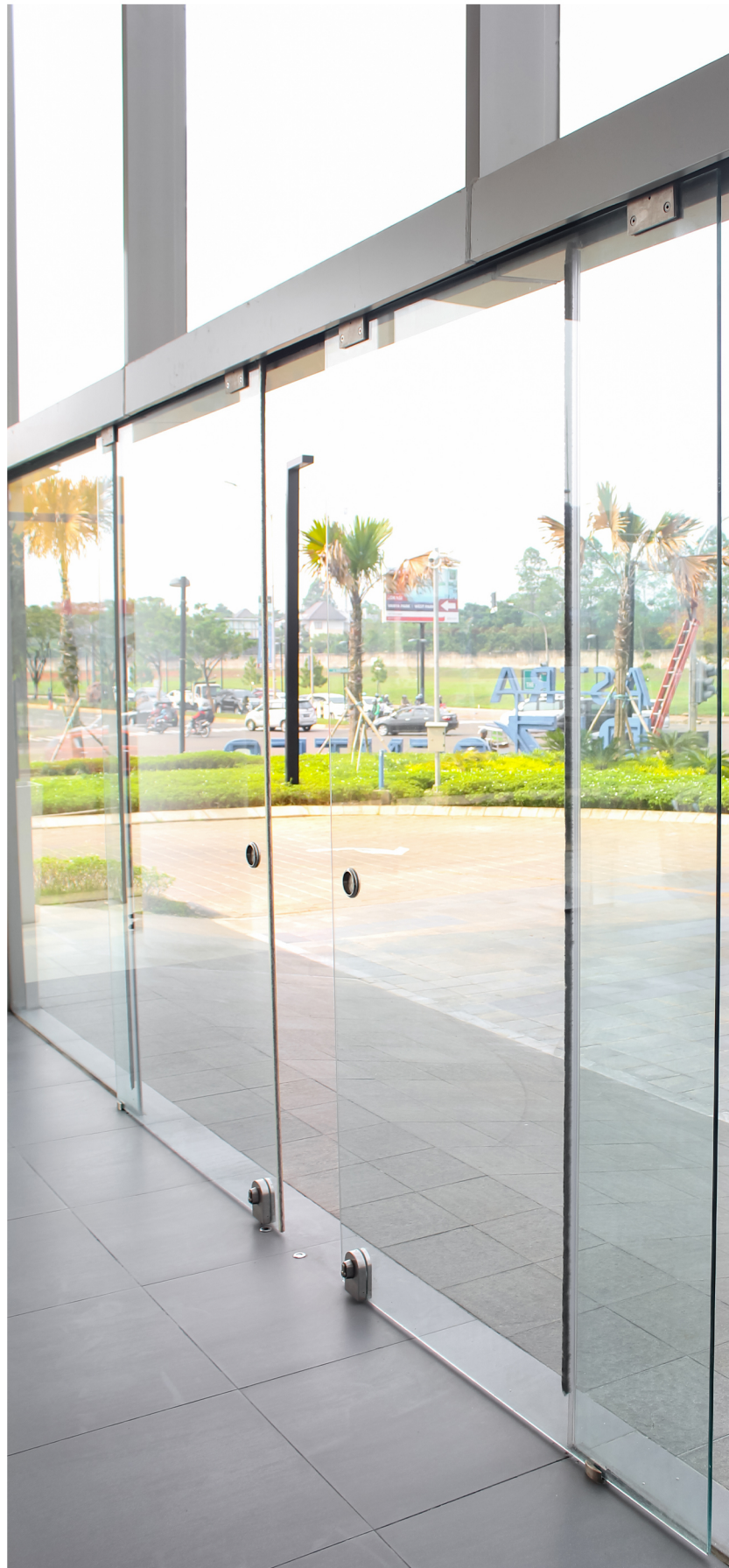
Project Showroom BMW BSD Serpong
